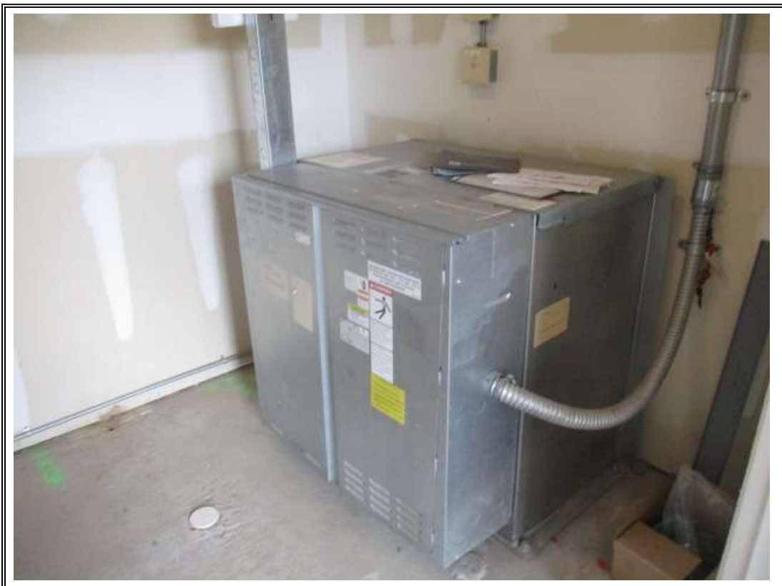
Photo 12: View of hydraulic elevator equipment.
